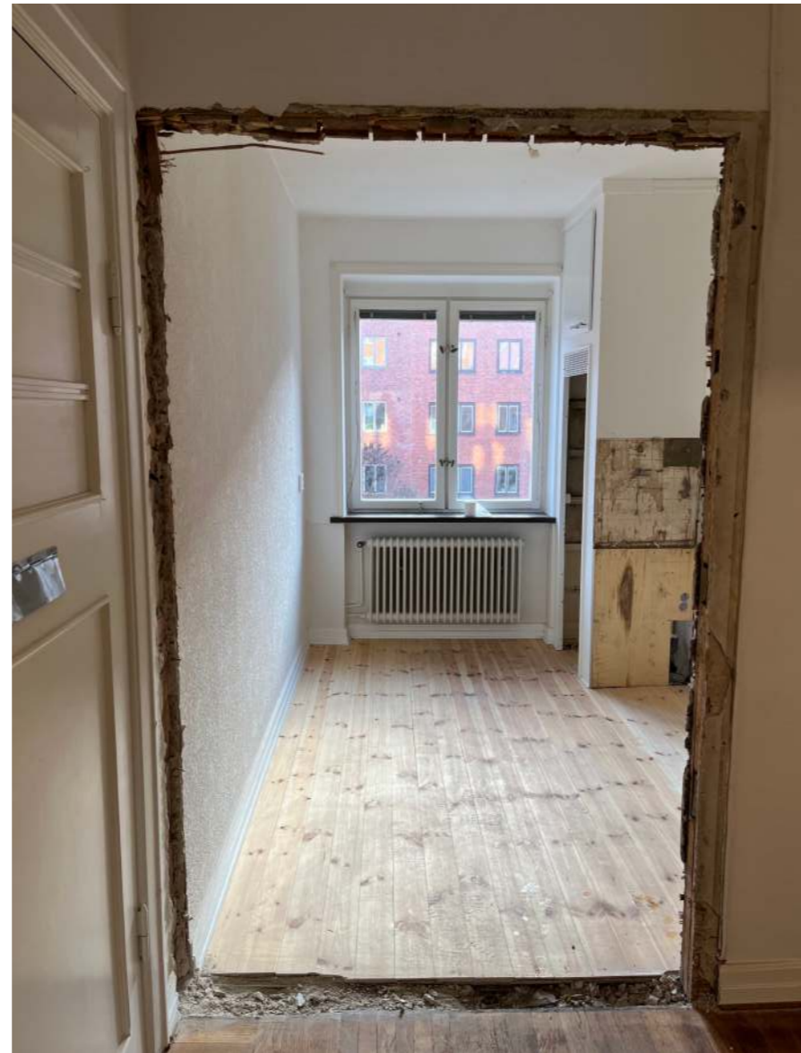
DEMOLITION PHOTO / EXISTING KITCHEN
