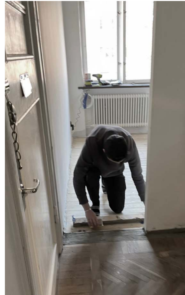
CASTING CONCRETE THRESHOLD TO BEDROOM
