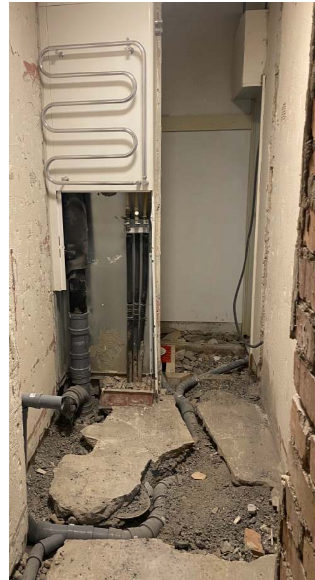
DEMOLITION PHOTO / EXISTING BATHROOM
